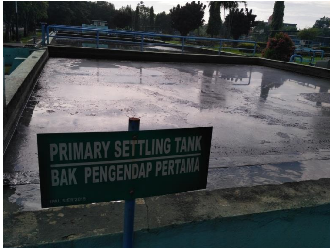
Gambar 5. Bak pengendap pertama ( Primary Settling Tank )
